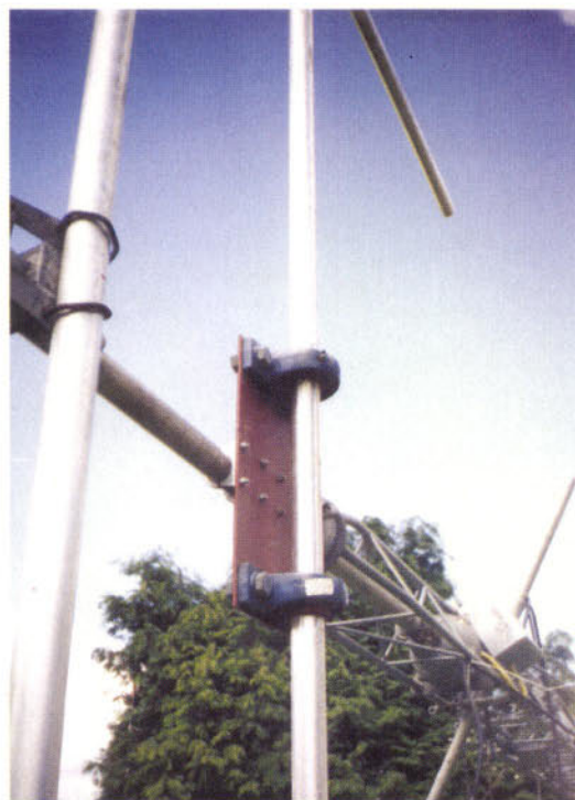
Fig. 4: A robust pivot bearing may be needed in some circumstances. See text for a slightly cheaper alternative that may be adequate for your needs.
